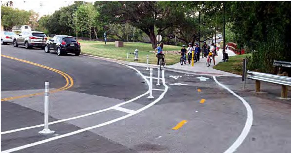
*A protected bike lane provides a connection to an existing sidewalk in Austin, TX<sup>88</sup>*
